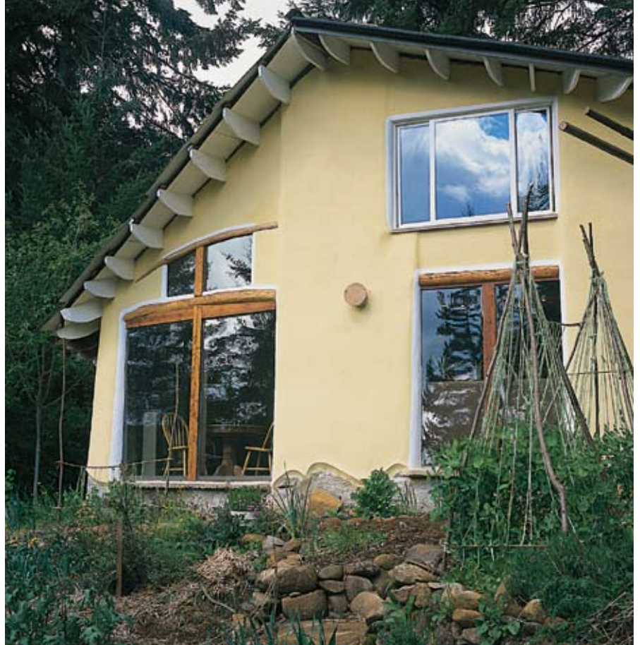
The couple framed the windows with salvaged lumber and used a lime plaster to add color to the exterior. The south-facing windows provide heat in the winter.
